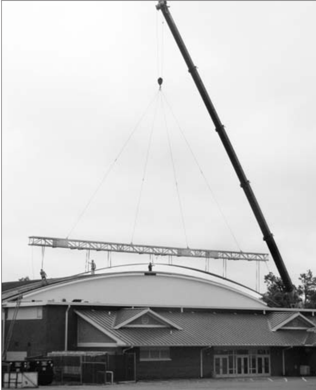
The large crane used by contractors to install metal on the roof of the middle school gymnasium last week was quite an attraction. The crane was extended to about 185 feet in order to lift into place 134-foot long seamless metal strips that went from gutter to gutter across the roof, according to Greg Binkley, school maintenance director. Swift Roofing of Murray is the contractor on the roofing project.
